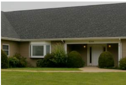
With no stairs leading to the entrance, this group residence in Brocton is an example of universal design.
